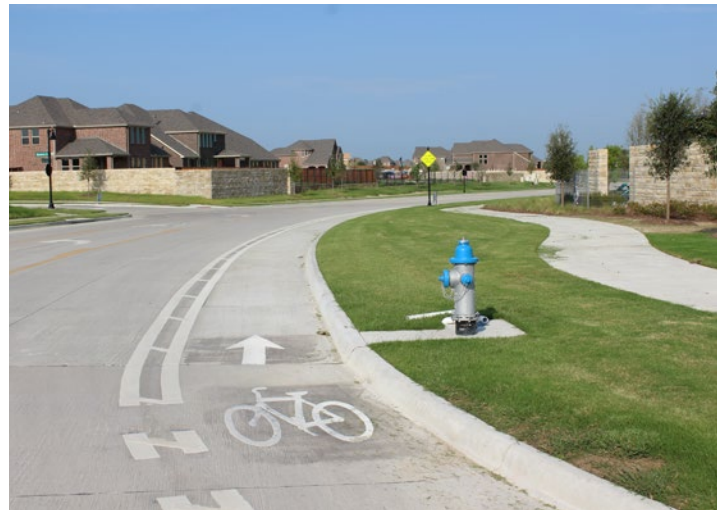
Picture 5: Excess pavement on Punk Carter Parkway has been re-stripped to implement the first bike lane in the city. (Source: Norris Design)
