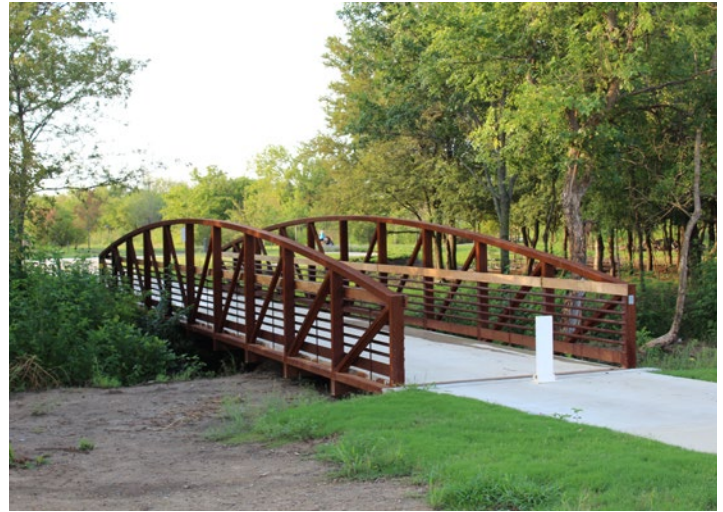
Picture 3: Quality infrastructure in place at Constellation Park in the Light Farms Development (Source: Norris Design)
