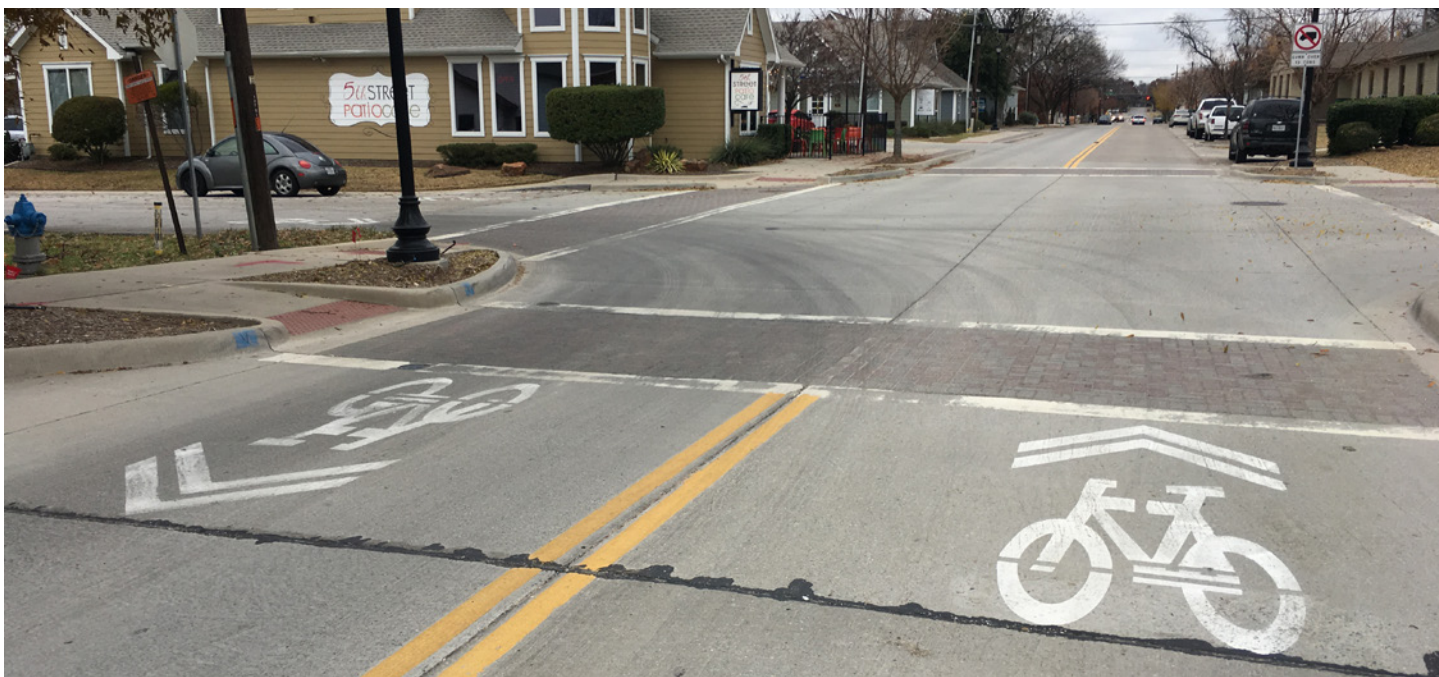
Pictured Above: Shared-lane markings identify where cyclists may commonly ride on a low-speed, low traffic volume street. (Source: Norris Design)
