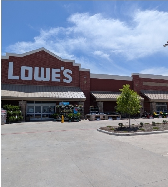
Lowe's - Celina, TX
