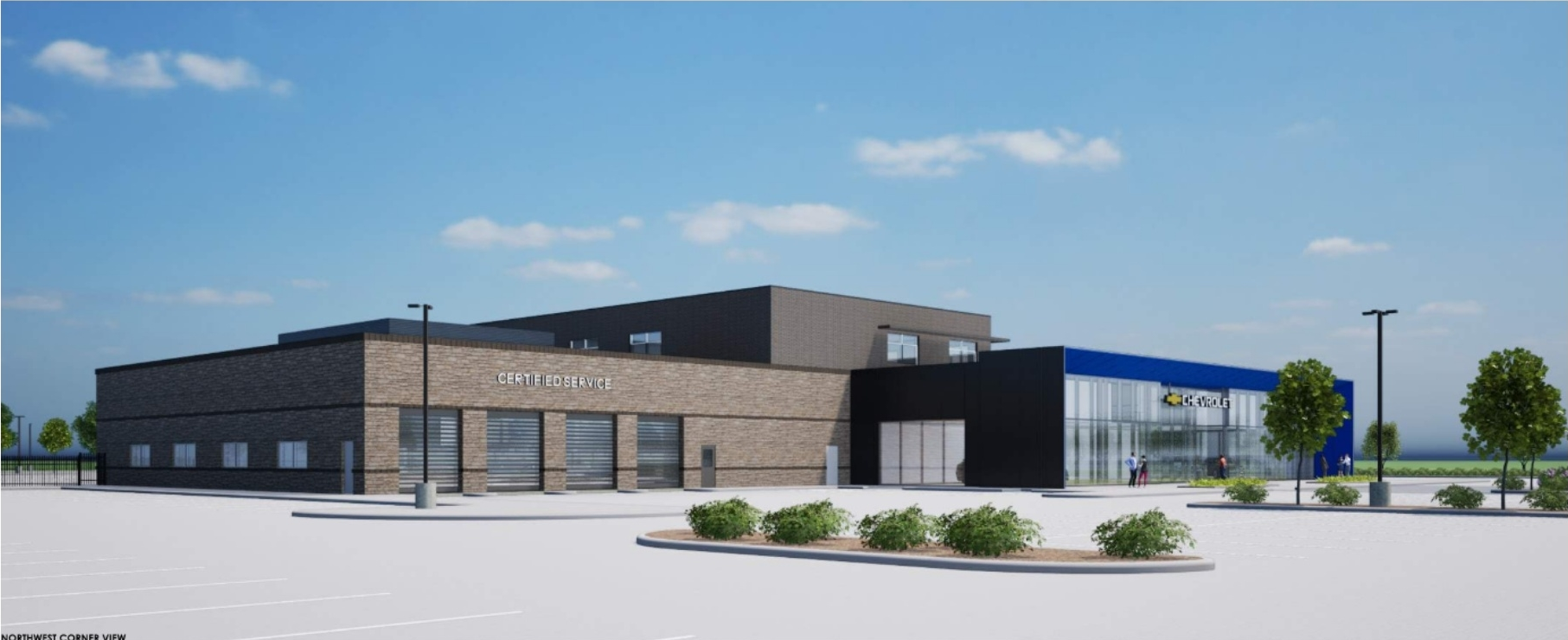
NORTHWEST CORNER VIEW
