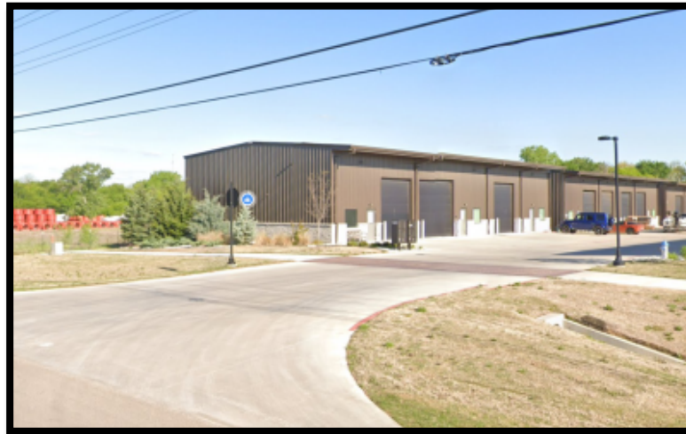
Masonry wainscot – not much better
