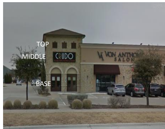
Examples of Tri-Partite Construction
