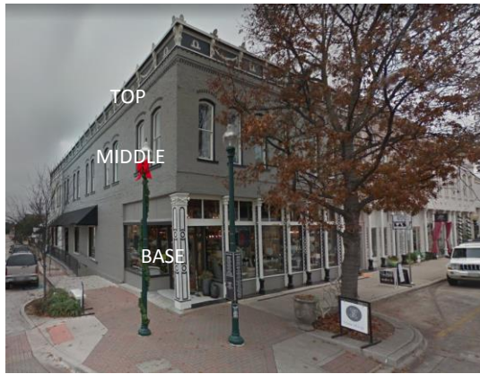
Examples of Tri-Partite Construction
