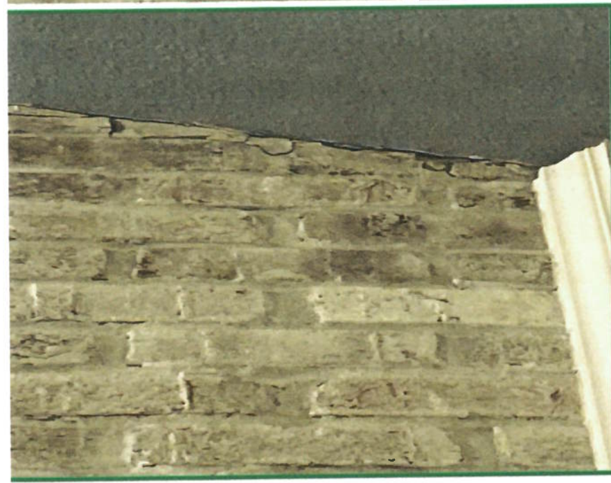
Top of fireplace Wall Damage, and Separation from the wall
