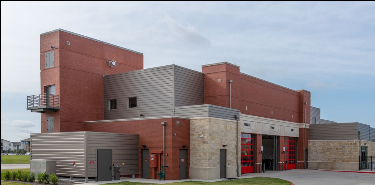
Anna Fire Station No. 2 – Original design
