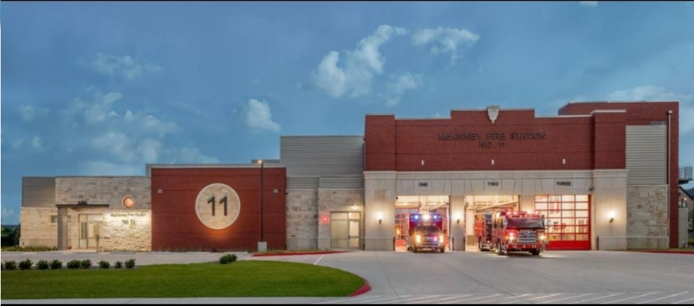
McKinney Fire Station No. 10 –
