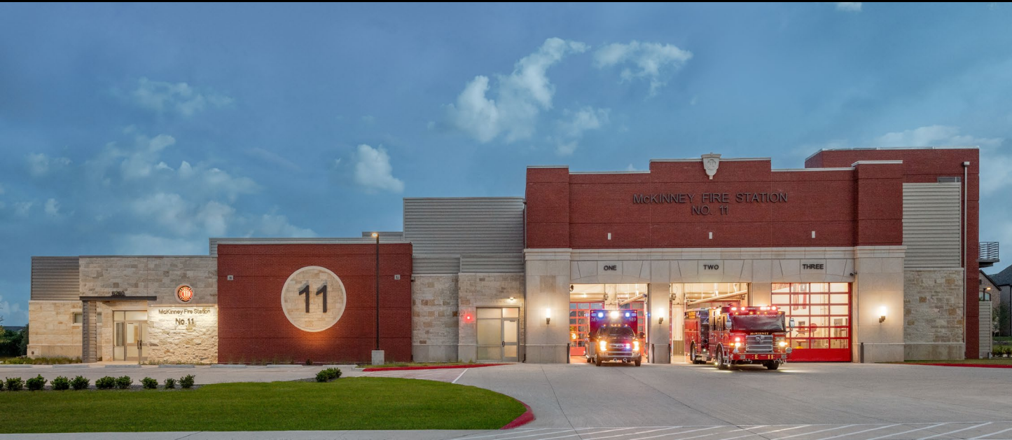
McKinney Fire Station No. 10 –
