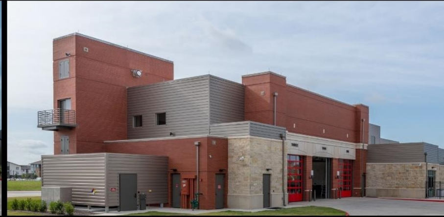
Anna Fire Station No. 2 – Original design
