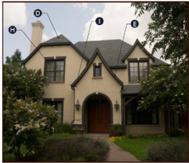
A>Prominent front-facing cross gable E>Nested gables C>Asymmetrical eaves D>Clipped gable E>Sweeping eaves F>Shed dormer G>Decorative half-timbering H>Gabled windows I>Brick or stone corbels
