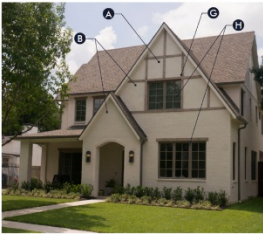
A>Prominent front-facing cross gable E>Nested gables C>Asymmetrical eaves D>Clipped gable E>Sweeping eaves F>Shed dormer G>Decorative half-timbering H>Gabled windows I>Brick or stone corbels
