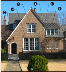
A>Prominent front-facing cross gable E>Nested gables C>Asymmetrical eaves D>Clipped gable E>Sweeping eaves F>Shed dormer G>Decorative half-timbering H>Gabled windows I>Brick or stone corbels
