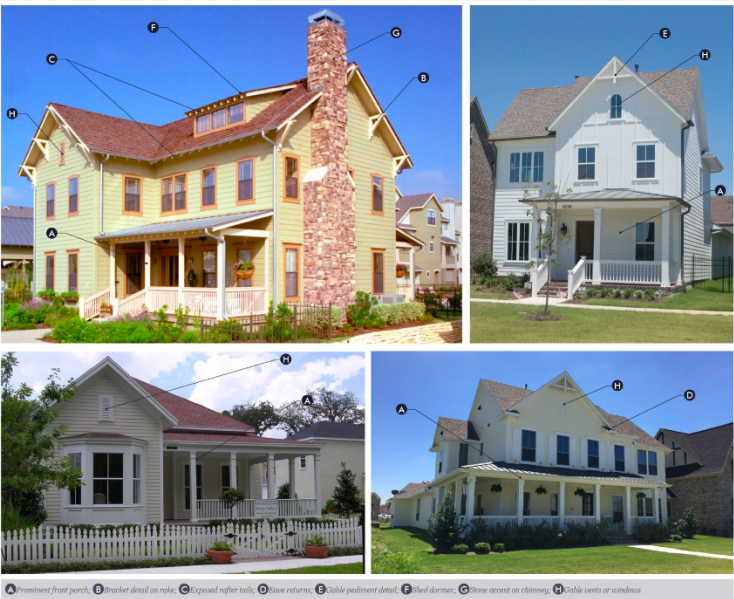
A: Prominent front porch; B: Bracket detail on rake; C: Gabled rafter tails; D: Gable returns; E: Gable pediment detail; F: Shed dormer; G: Stone accent on chimney; H: Sash vents or windows
