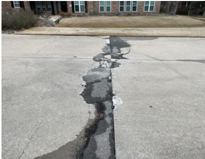
Concrete Panel Replacement
