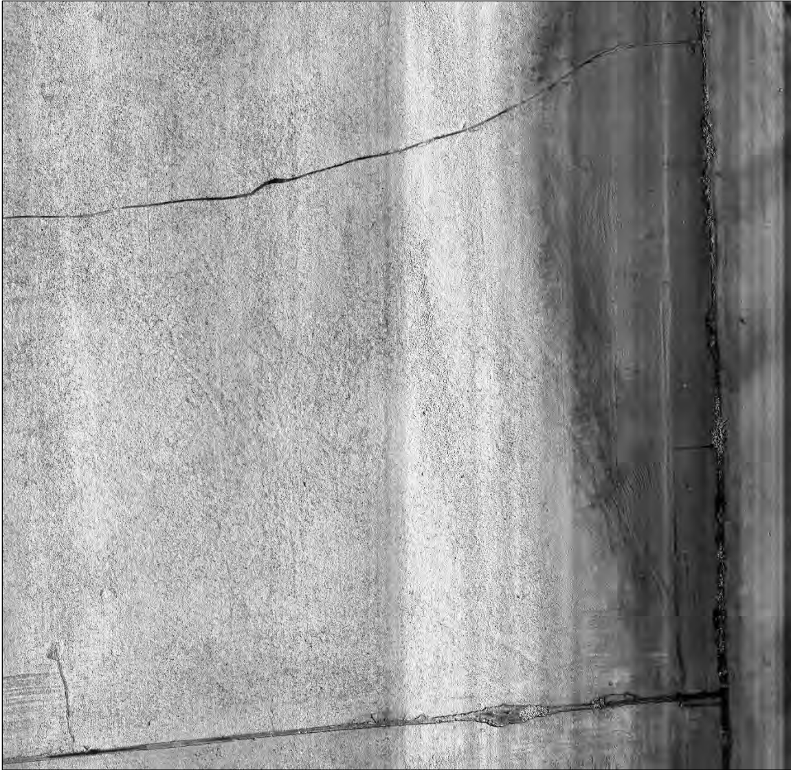
Figure 7: Pavement Image Example
